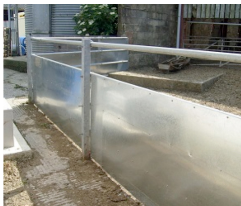
Fig.1: Galvanised steel panels on yard fence
